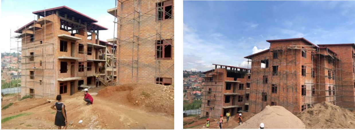
Figure 24: Photos of the project under construction
