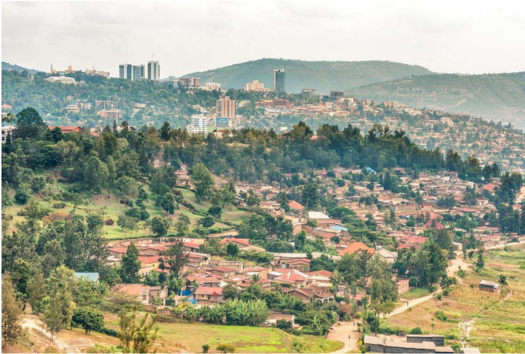
Figure 7: Lower density housing in Kigali
